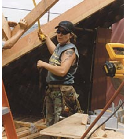
Charlene Getchell of Getchell Construction
